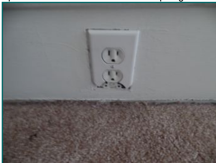
Broken cover plate.
