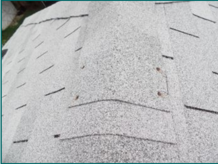
Exposed roofing nails.
