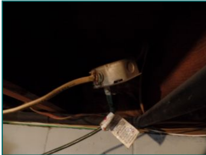
Loose junction box in basement.
