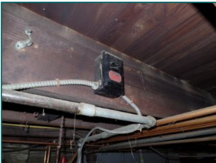
Location: Boiler emergency shut off switch.
