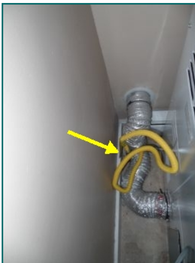
Location: Dryer gas shut off valve.
