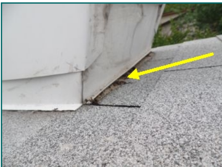
Chimney flashing
