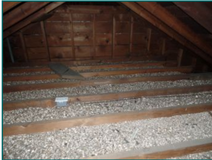
Vermiculite insulation.
