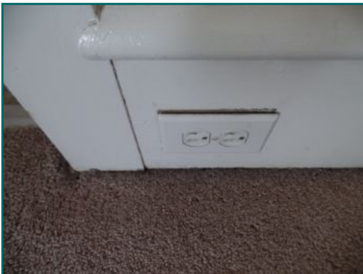
Open ground/ loose receptacle.
