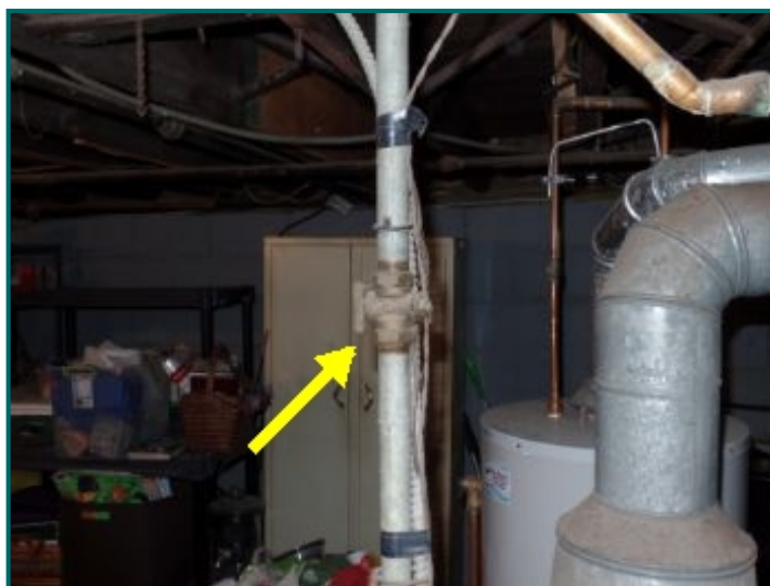
Boiler gas shut off valve.
