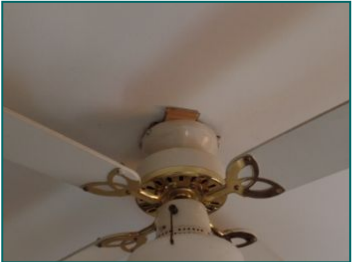
Fixture not properly secured.
