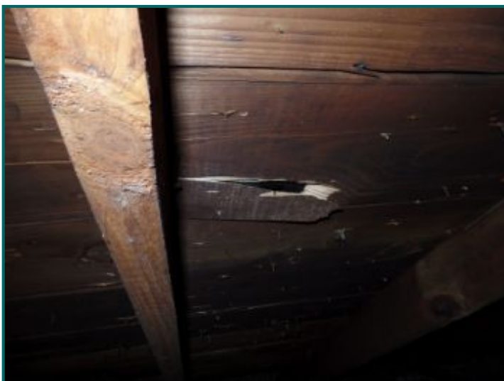
Damaged roof sheathing.
