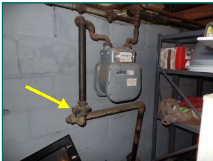
Gas meter and main shut off location.
