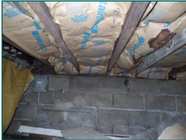
Vapor barrier incorrectly installed.
