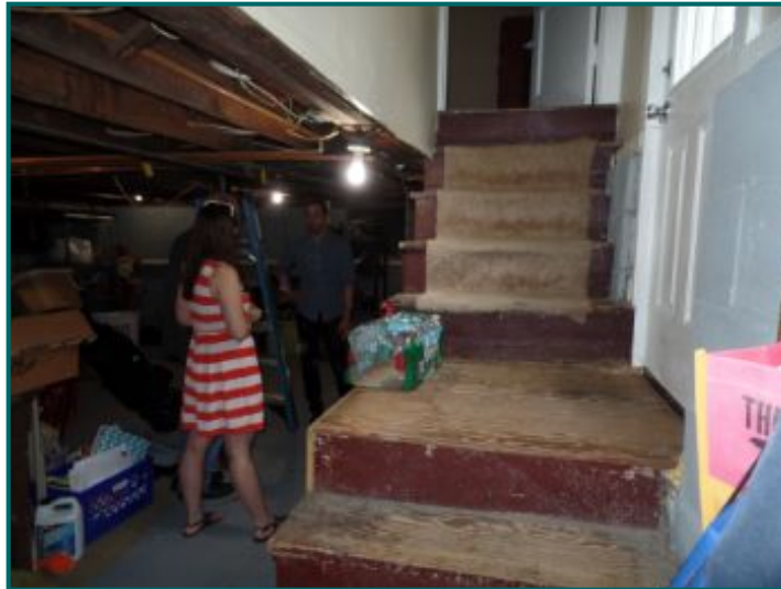
No safety handrail or guard rails.
