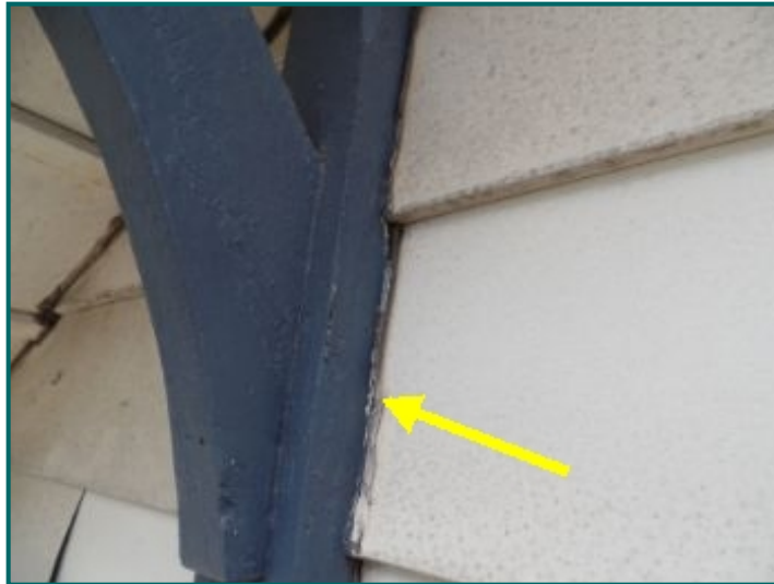
Caulking maintenance required.
