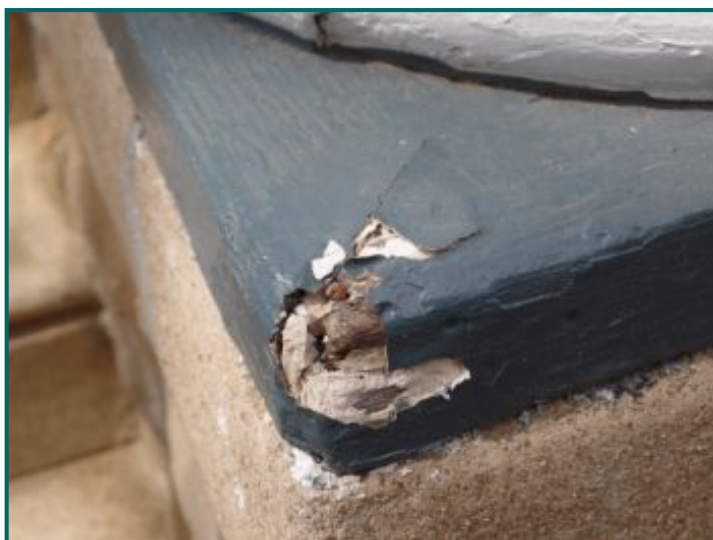
Moisture damage at column base.
