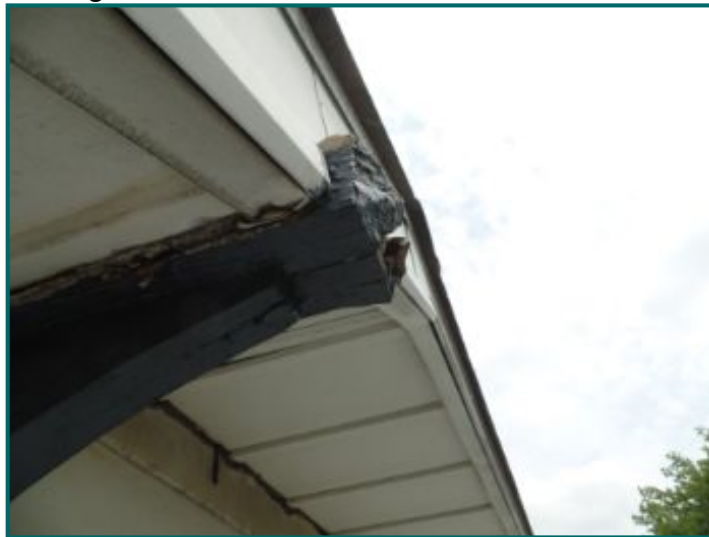
Damage at outrigger ends.
