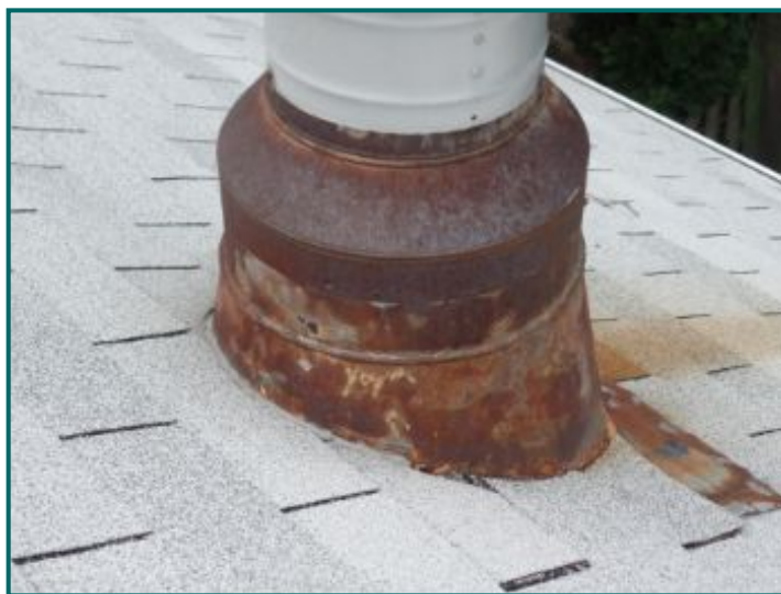
Rusted turbine vent.
