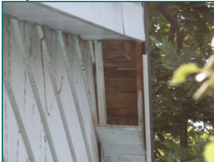
Missing soffit panel.
