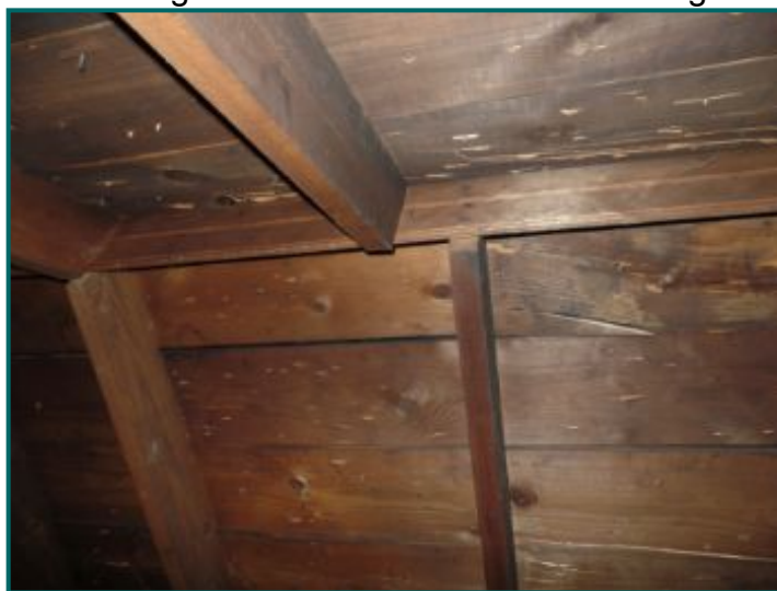
Offset roof rafters.
