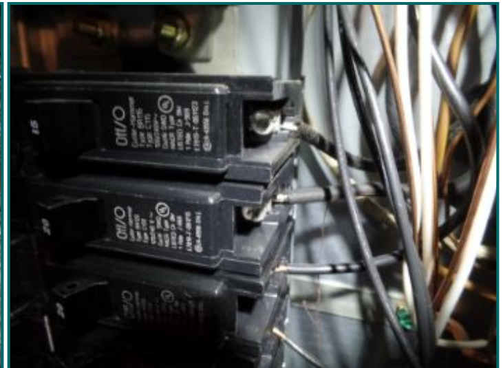
Solid aluminum wiring.
