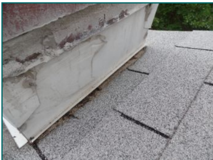
Chimney flashing.
