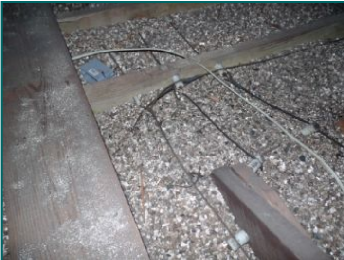
Live knob & tube wiring.
