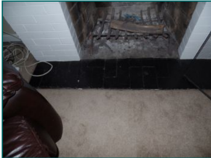
Inadequate hearth extension.
