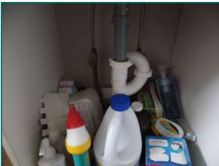
"S" trap, first floor 1/2 bath.
