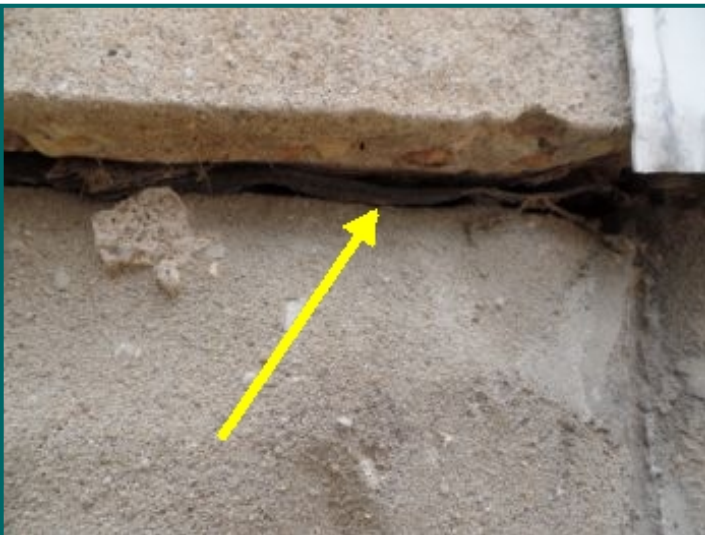
Recommend sealing all masonry joints.
