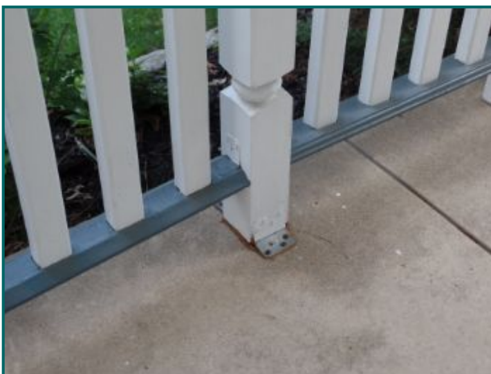
Loose center guardrail post.
