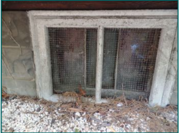
Wood/soil contact at basement window.
