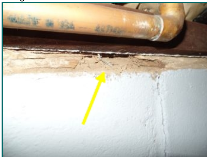
Insect damage at sill plate.
