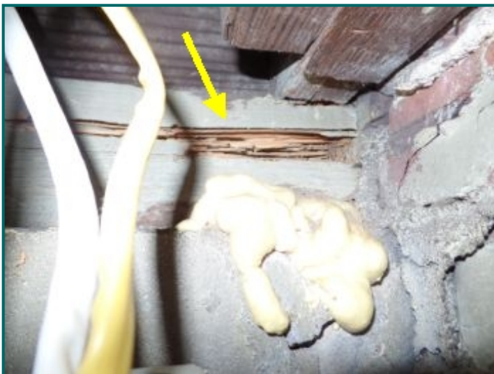
Insect damage at sill plate.
